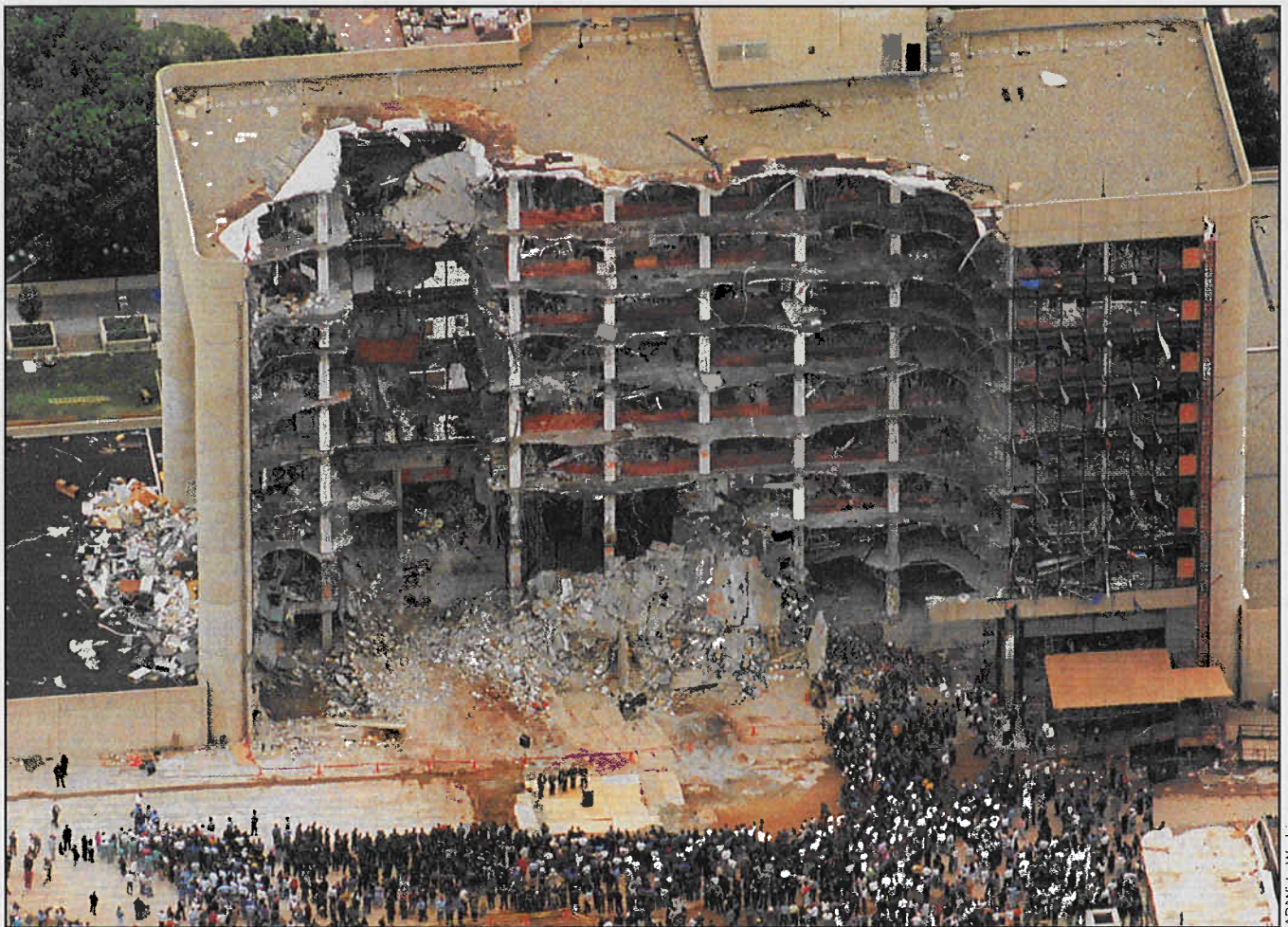
Aerial view of bombed-out Alfred P. Murrah Federal Building (above) provides reference point for General Partin's "Tab 2" diagram of building damage (below). The concentric rings radiating out from the bomb show the roughly equal levels of damage potential and the rapid dissipation of the blast wave pressure as it moves out from the source.
